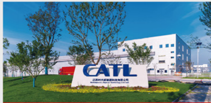
CATL Liyang Facility New Production Facility in Thuringia (under construction)
